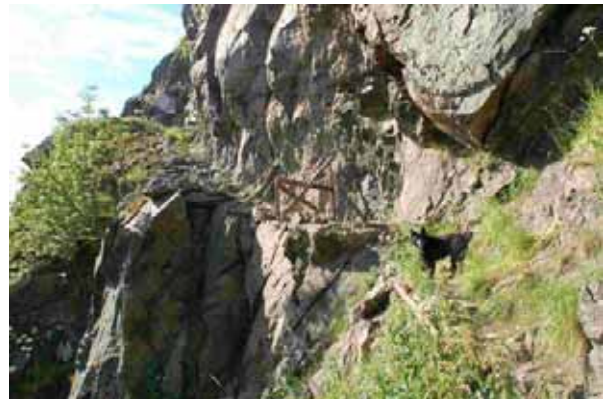
Figur 11 Grinda treng utskifting.
